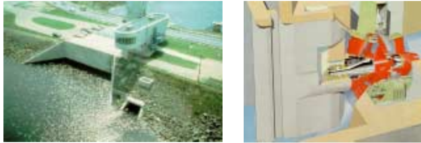
Figure 2-4 Annapolis Royal tidal plant (Sulzer Technical Review, 1987)
